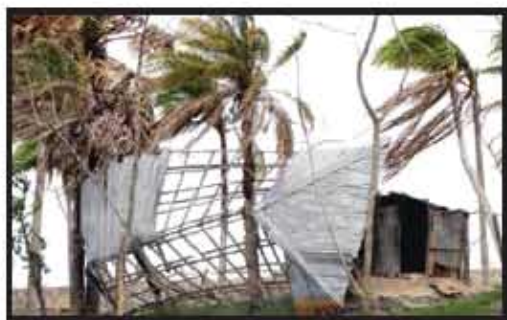
The wind is blowing the roof away.
