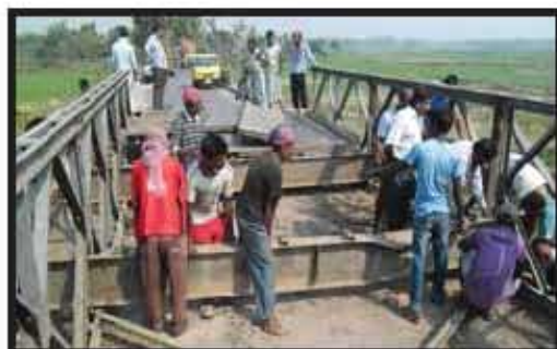
The workers are repairing the bridge.
