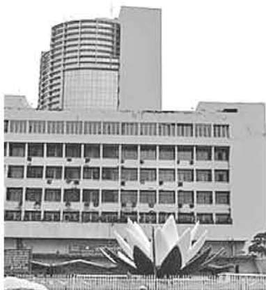
Sonali Bank Building
