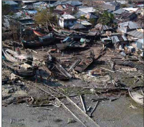
Damage from cyclone
