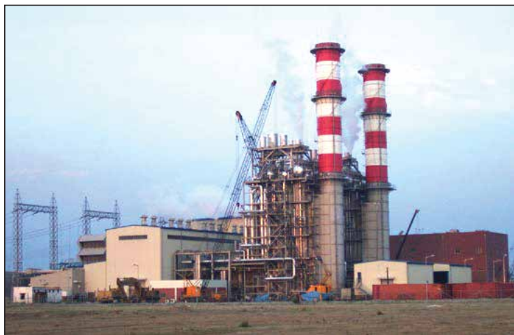
A power plant of Bangladesh
