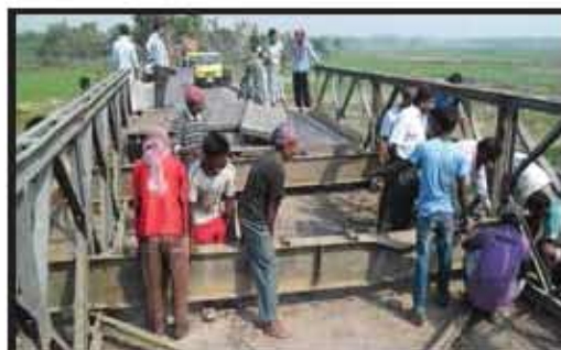
The workers are repairing the bridge.
