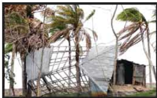
The wind is blowing the roof away.
