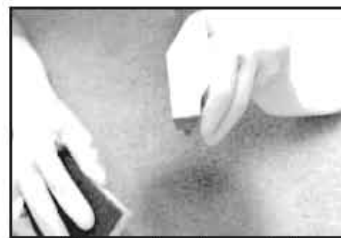
Removing iron stain
