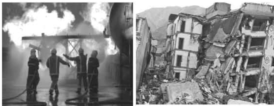
Picture: Damages from fire and earthquake.
